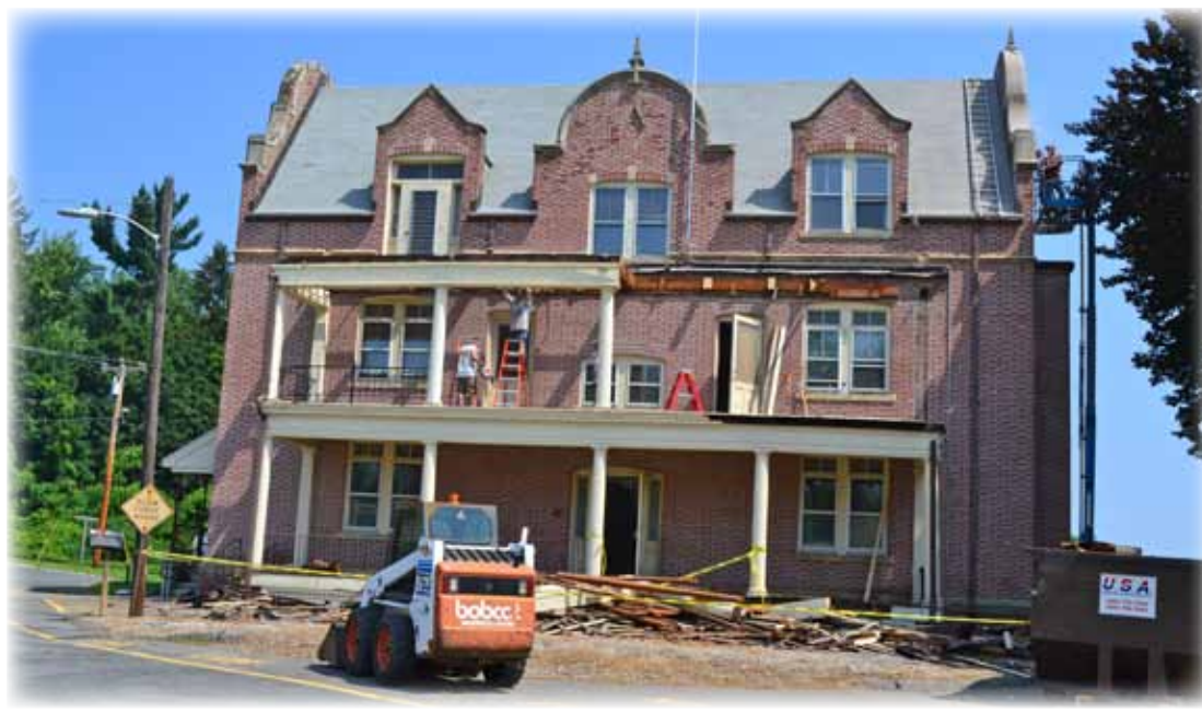
Work in progress at McCleary Manor.
